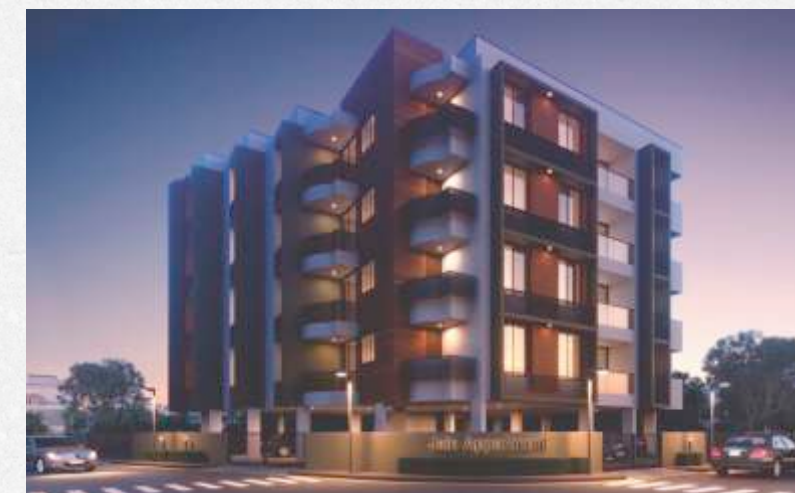
JAIN APARTMENT - COMPLETED
