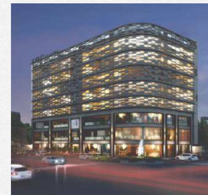
SCARLET BUSINESS HUB - COMPLETED
