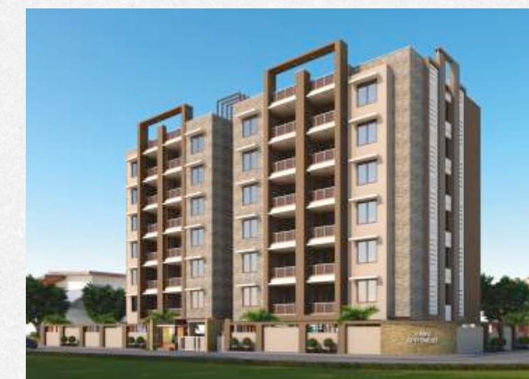
VIMAL APARTMENT - COMPLETED
